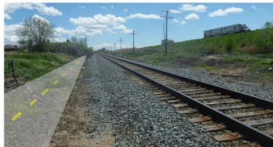
Figure 3-9. The FrontRunner Trail would follow the current route of the Union Pacific railway between South Willard and Brigham City.
